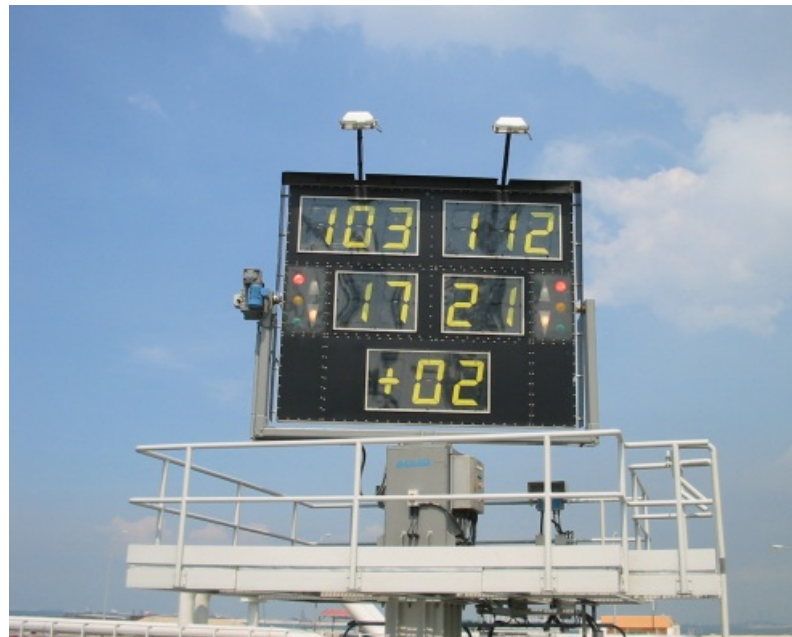
A jetty-mounted large digit display from Strainstall, providing interested parties with the relevant berthing parameters
