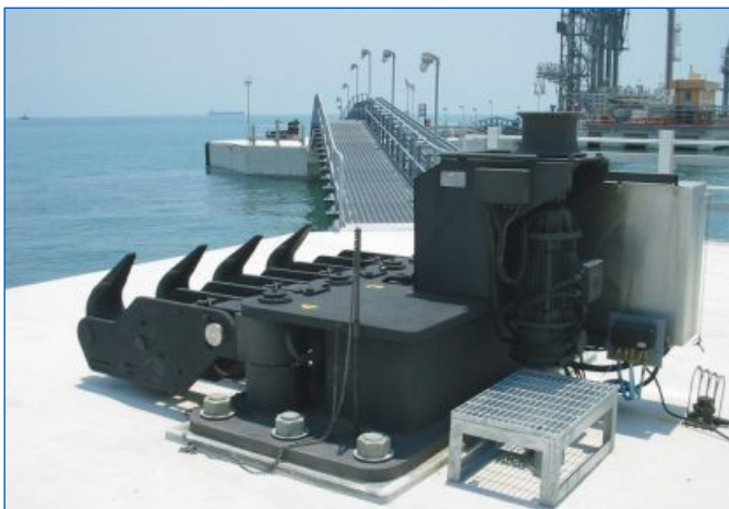
Figure 1. Jetty fitted with quick release mooring hooks.
